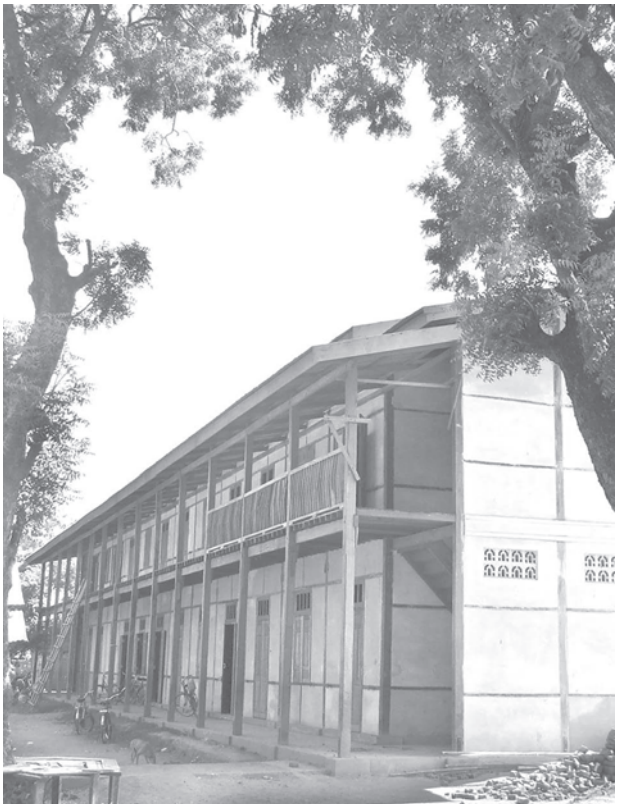
Photo shows a two-storey new building at Nay Pyi Taw Tatkon BEHS No. 1.
