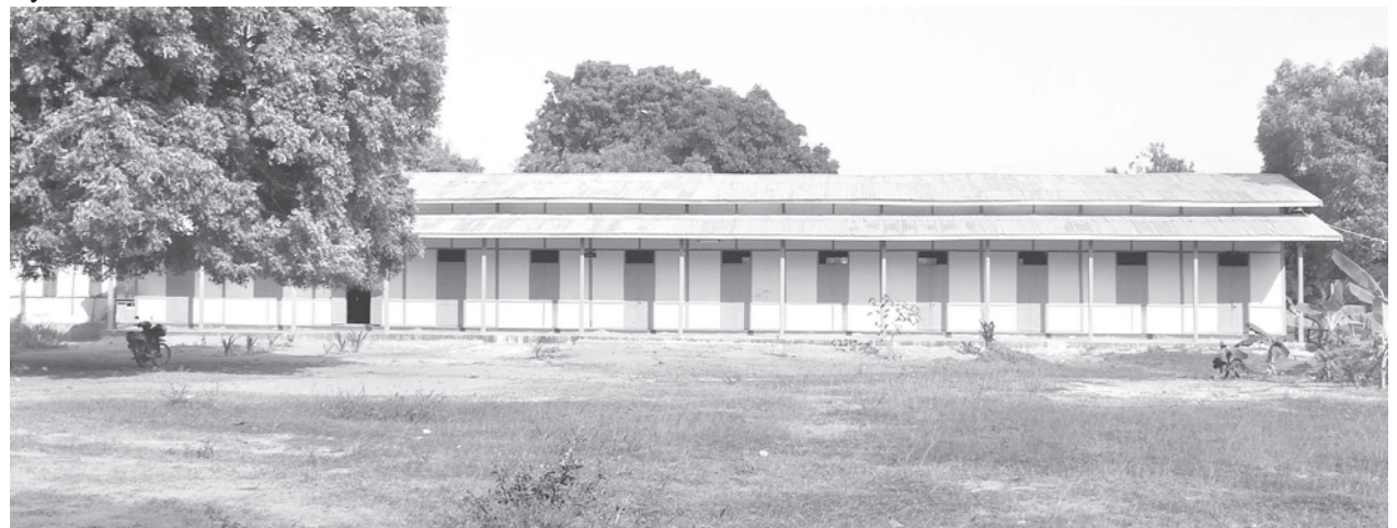
One-storey building of Nay Pyi Taw Tatkon BEMS (Nyaunglunt).
