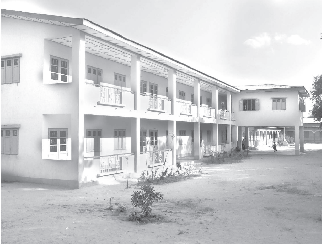
A two-storey building of Magyibin Basic Education Middle School (Branch) in Nay Pyi Taw Tatkon.
