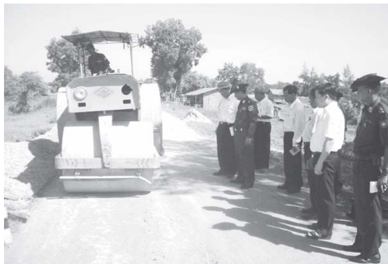
Minister Maj-Gen Khin Maung Myint inspects roadworks on Yangon-Pathein road. CONSTRUCTION
