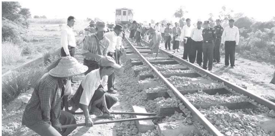
Minister Maj-Gen Aung Min inspects Pyawbwe-Natmauk-Magway railroad construction project.—MNA
