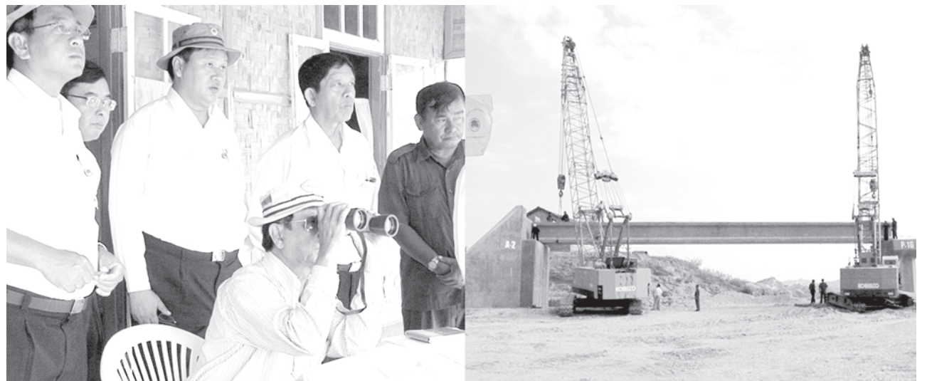
Deputy Minister for Construction U Tint Swe inspects Yaw creek bridge (Railway) construction project.—MNA
