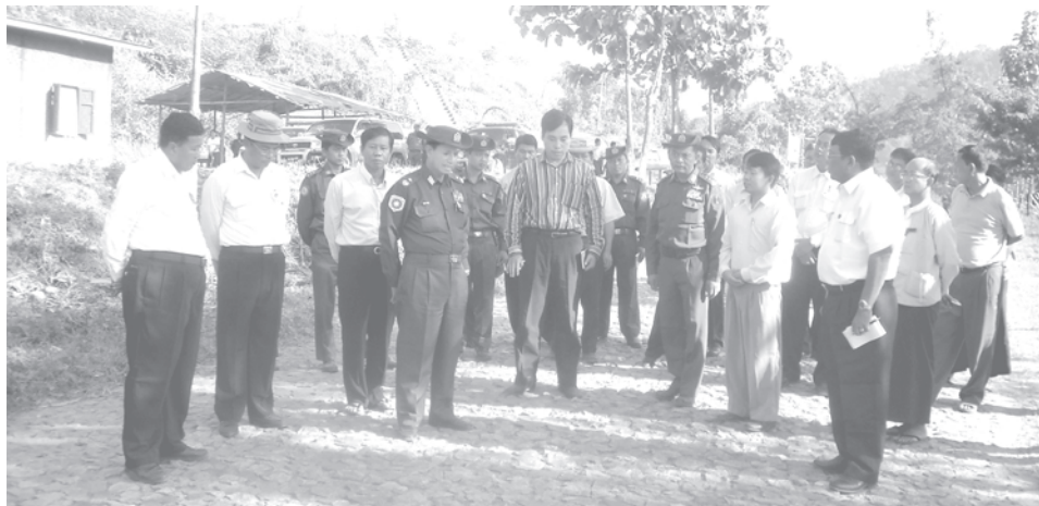
Minister Maj-Gen Khin Maung Myint inspects placing of gravel along Bhamo-Myitkyina road.—MNA
