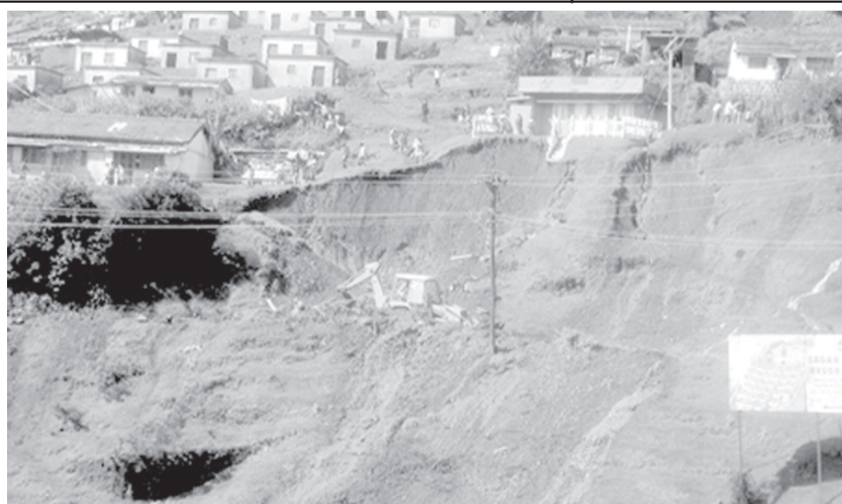
This photo taken on 11 Nov, 2009 shows the scene of the landslide in Nilgiris district of Tamil Nadu, southern state of India. The massive landslide took place here on Wednesday has killed 43 people and left nearly 100 others wounded.—XINHUA
