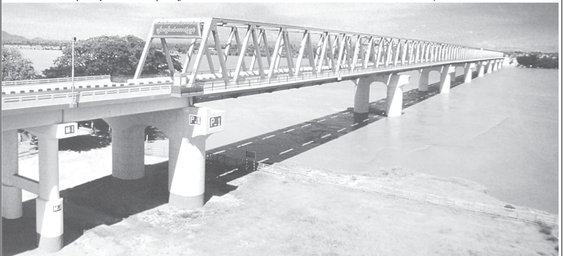
Photo shows Chindwin Bridge (Monywa), vital for regional development and border trade.
