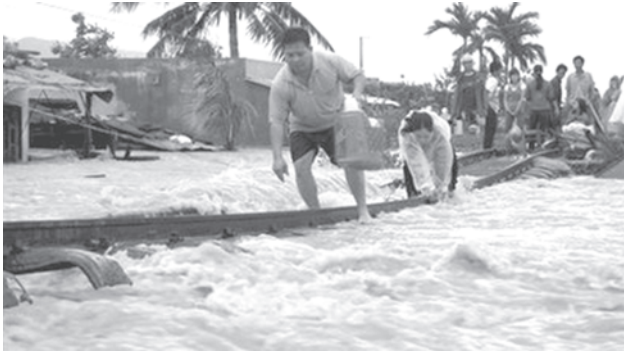
People are seen negotiating a flooded railway in the central Vietnamese province of Binh Dinh, a few days ago, after the passage of tropical storm Mirinae. At least 13 people have been killed in a landslide in central Vietnam following storms and flooding that have now left almost 130 people dead, according to officials.—INTERNET
