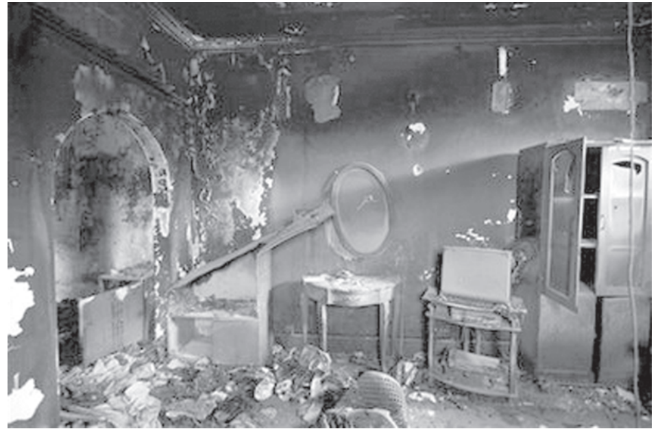
A burned down room is seen in the destroyed guesthouse that left five UN staffers dead in Kabul, Afghanistan, on 5 Nov, 2009. The United Nations said on Thursday that it is temporarily relocating more than half its international staff in Afghanistan following last week's deadly Taliban attack against UN workers, the most direct targeting of its employees during decades of work in the country.—INTERNET
