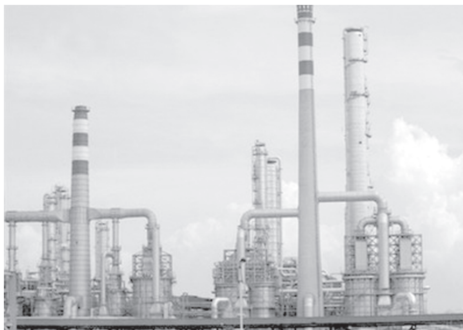
A chemical plant of Chinese energy giant CNOOC and Anglo-Dutch firm Shell petrochemical plant in Daya Bay in southern China.—INTERNET
