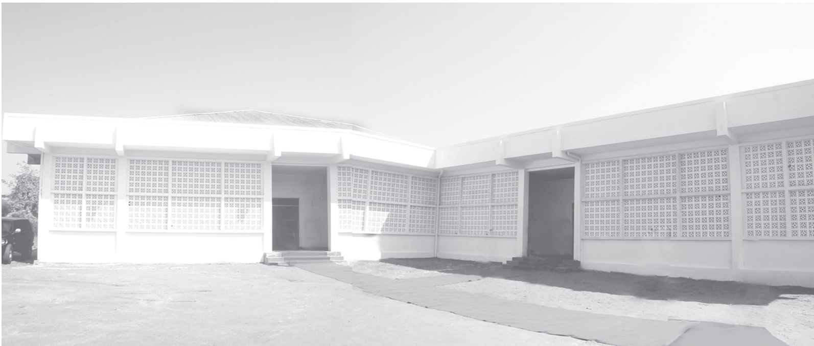
Photo shows extended 200-bed hospital of Pyapon.—MNA
