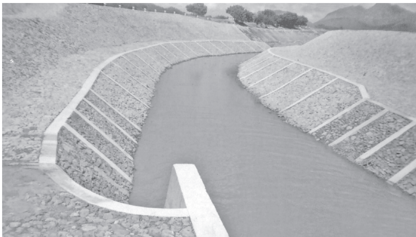
The main canal of Myogyi Diversion Weir.
