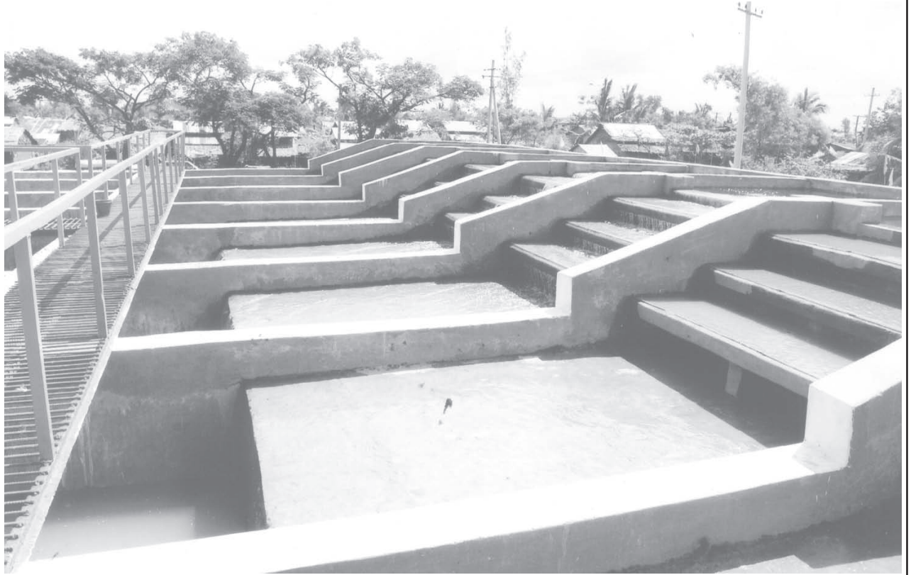
Massive structures for purifying water seen at water supply station No. 1+2 in Dagon Myothit (South) Township.
