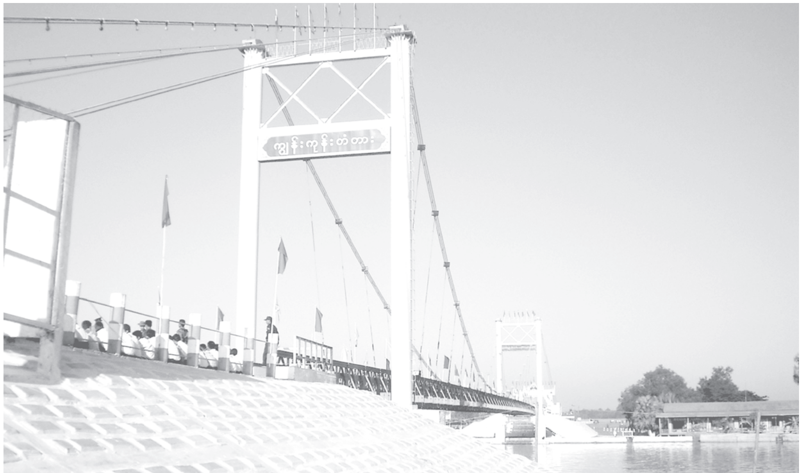
Kyungon Bridge in Wakema Township.
