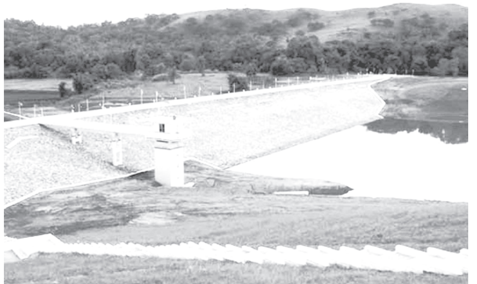
Phayagon dam in Taunggyi Township, Shan State (South).
