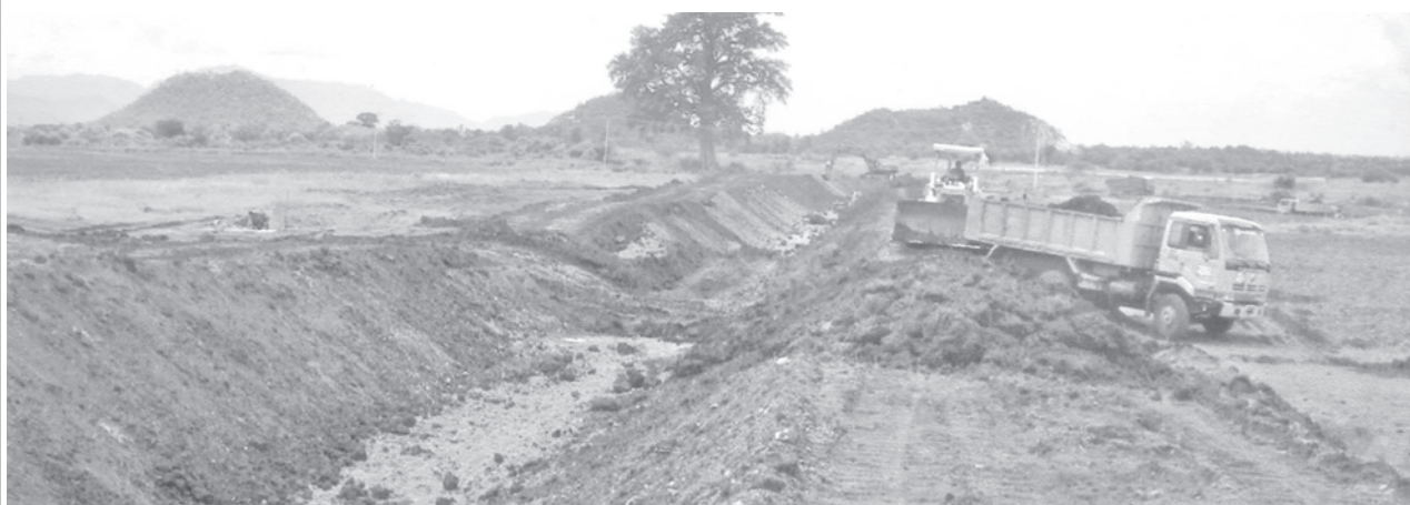
Groundwork is carried out with tipper lorries.
