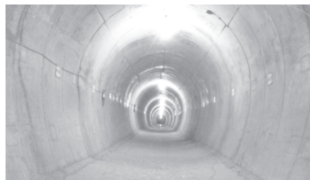
The inner part of the diversion tunnel under construction.
