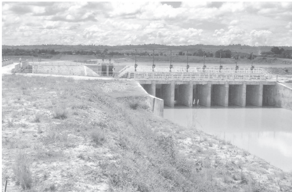
Eight left valves seen at Yenwe Diversion Weir.
