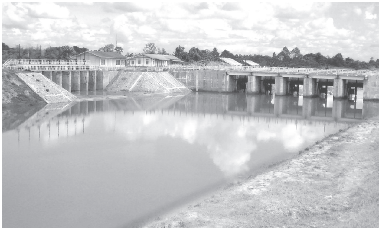
Photo shows Yenwe Diversion Weir in Kyaukdaga Township.
