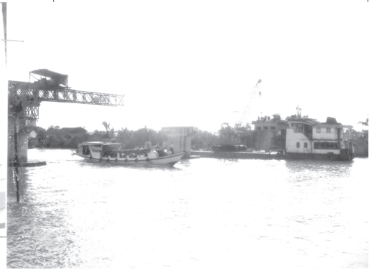
Commander Maj-Gen Kyaw Swe inspects the construction of Rasudine Bridge No-2 on the Maubin-Shwetaunghmaw-Kyaikpi-Mawlamyinegyun Road.—MNA
