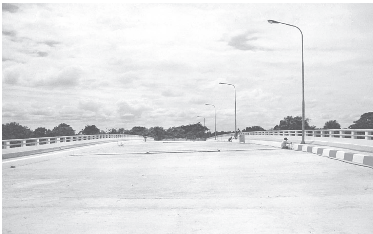
Overlay RC type truss.
