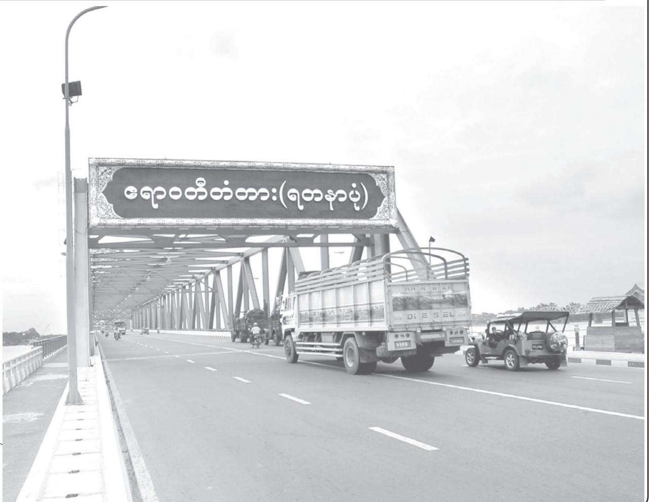
Vehicles passing through Ayeyawady Bridge (Yadanabon).
