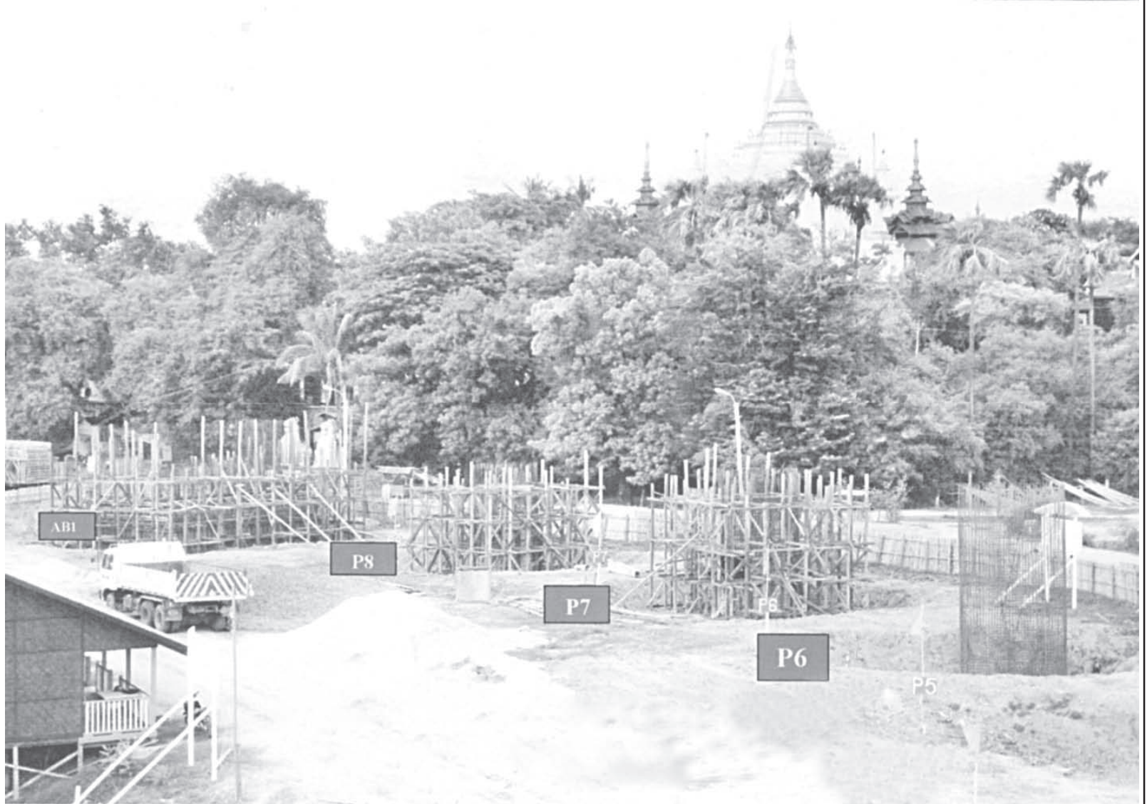
Site of extended upward approach bridge on Mandalay bank.
