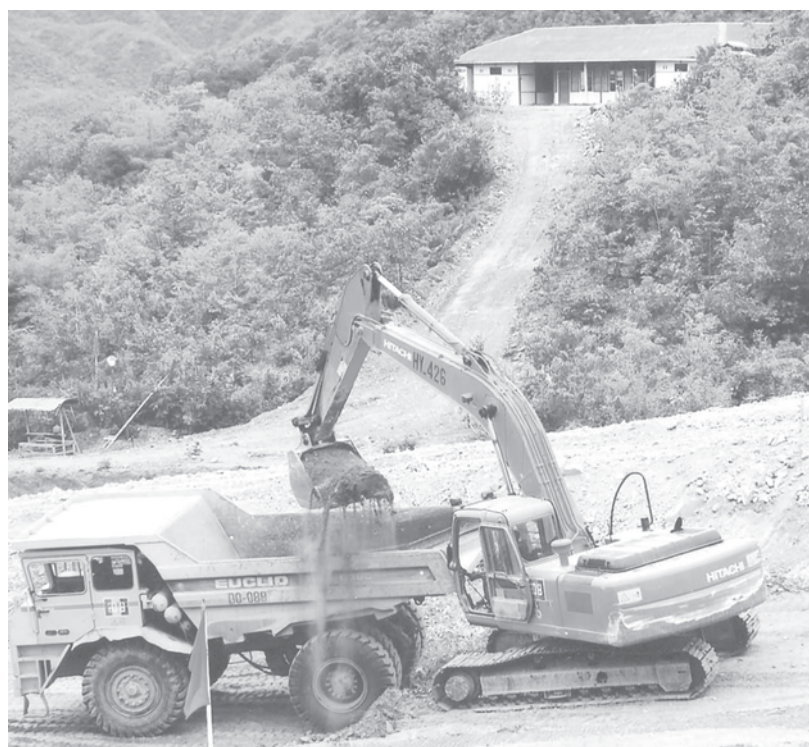
Heavy machinery at work at construction site of Myogyi Dam.
