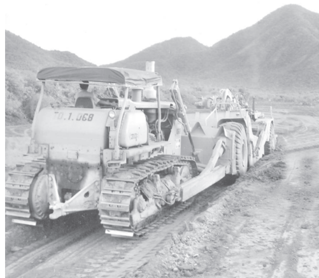
Heavy machinery being used for ground work of Myogyi Dam.
