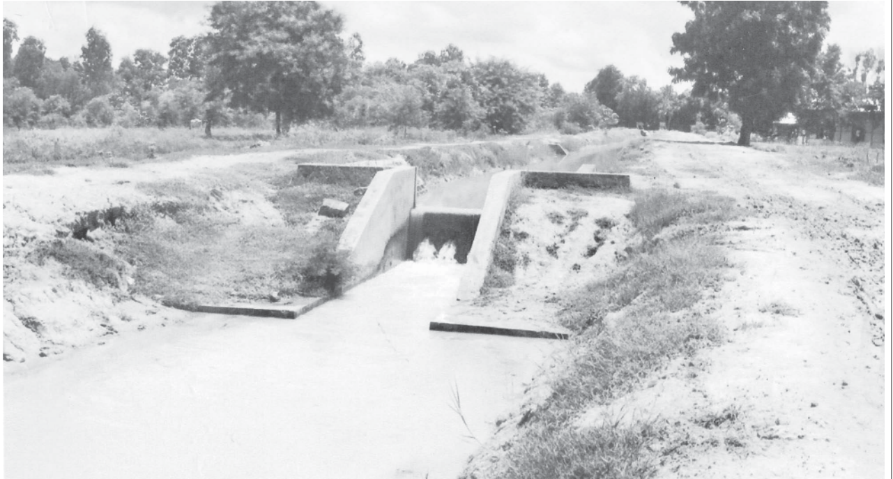
Feeder canal No. 2 of Yanpei Dam supplying water to 800 extended acres of land in Taungdwingyi Township.
