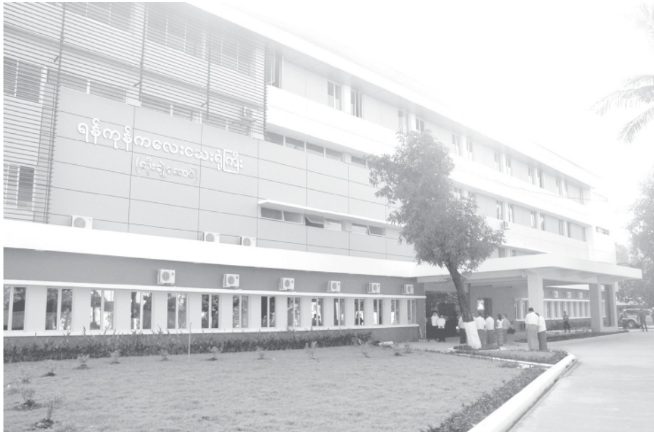
Photo shows new building of Yangon Children's Hospital.—MNA
