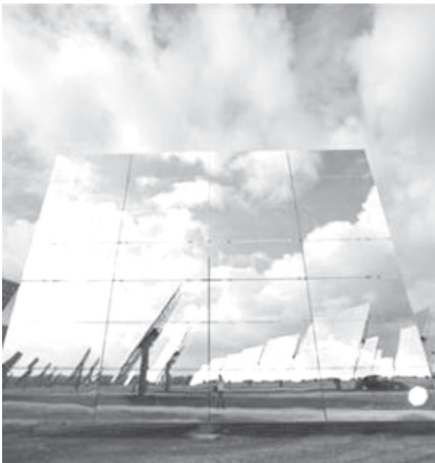
A general view of the new PS20 solar plant which was inaugurated last month at "Solucar" solar park in Sanlucar La Mayor, near Seville, on 7 October, 2009. The solar thermal power plant uses mirrors to concentrate the sun's rays onto towers where they produce steam to drive a turbine, producing electricity. —INTERNET
