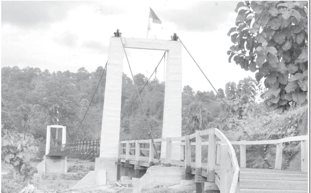
Ma Sein-Kyauk Sin suspension bridge in Kalewa.
