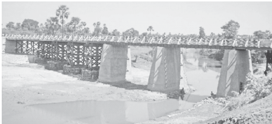
Gabarte Bridge on Meiktila Township section of No (1) Inter-District Road.
