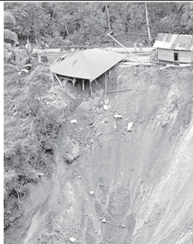
An aerial picture shows a damaged house on top of the landslide area in Pariaman. Indonesia called off the search for survivors in the quake-hit city of Padang on Monday as officials sought to contain the risk of disease caused by thousands of trapped bodies.—INTERNET
