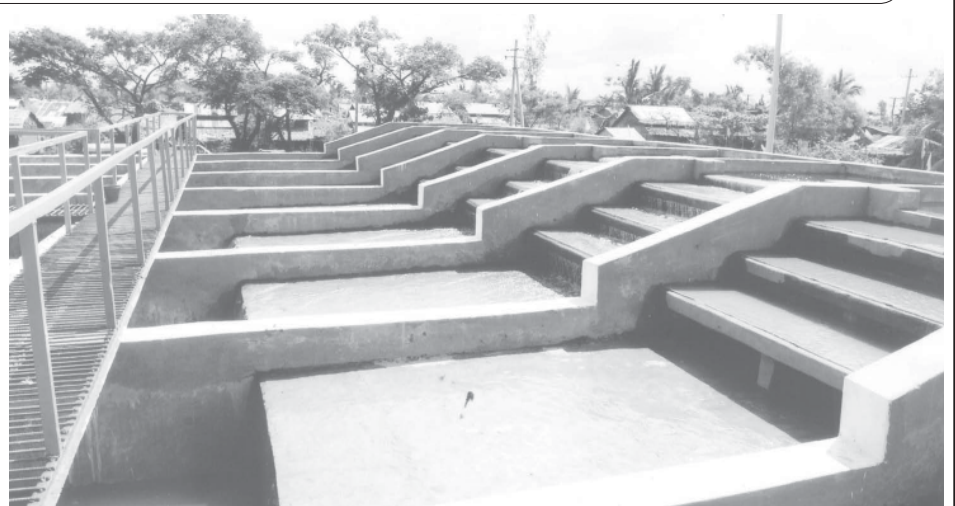
Filtering tanks of the water supply station in Dagon Myothit (South) Township.
