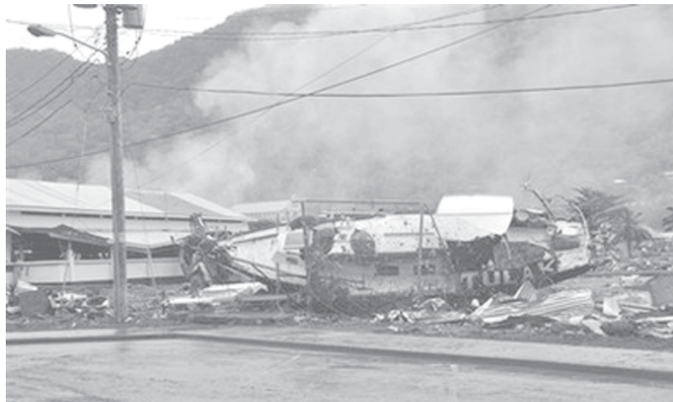
A boat is aground beside a street on 1 Oct, 2009 in Pago Pago, American Samoa after a tsunami struck the island on 29 Sept, 2009 and carried it away from the harbour. The tsunami also caused structural damage to buildings and deposited mounds of debris.—INTERNET
