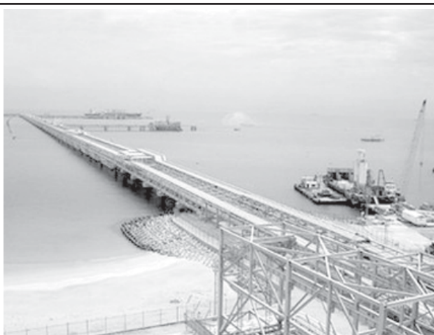
The largest and most advanced pier in the Middle East at Kuwait's largest refinery of Al-Ahmadi just north of Al-Shuaiba.
