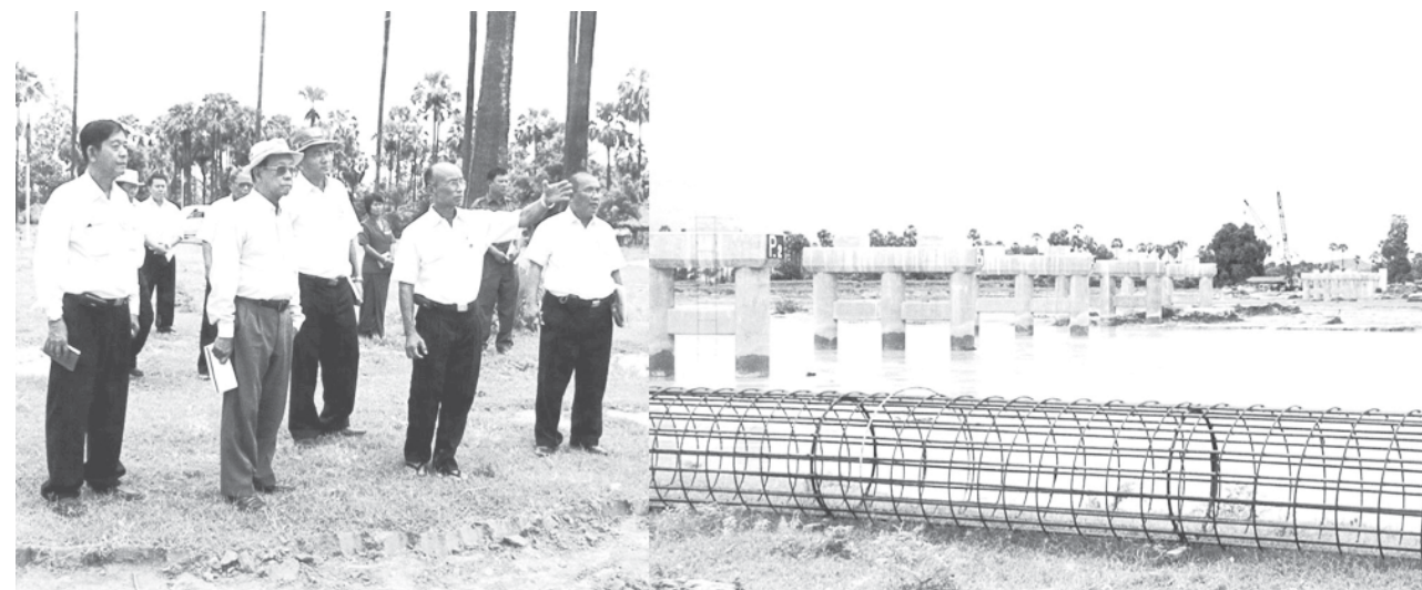
Deputy Minister U Tint Swe inspects Myaukyama creek bridge construction project.—CONSTRUCTION
