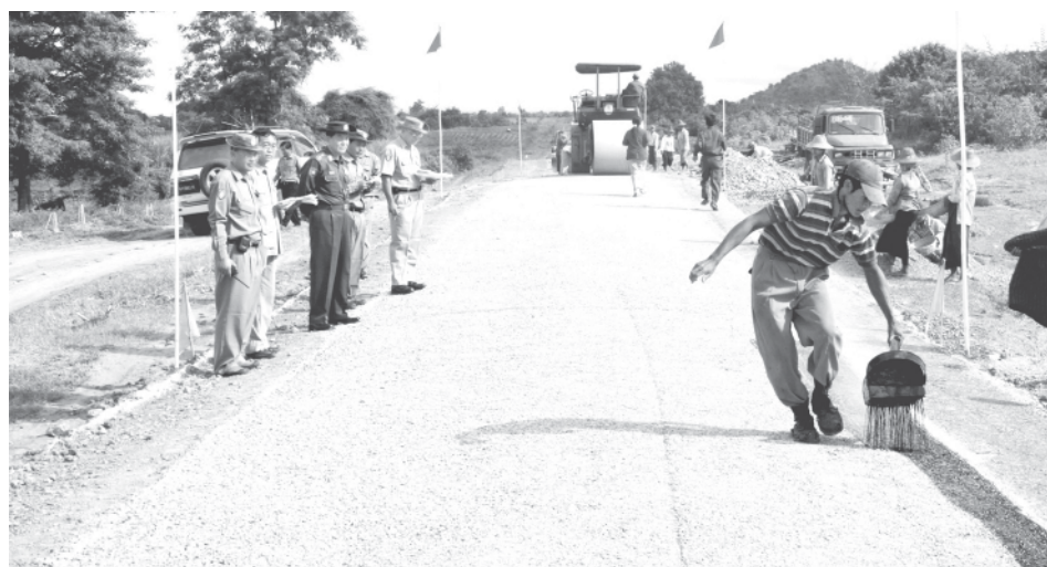
Minister Col Thein Nyunt inspects roadworks in Yamethin Township. —MNA
