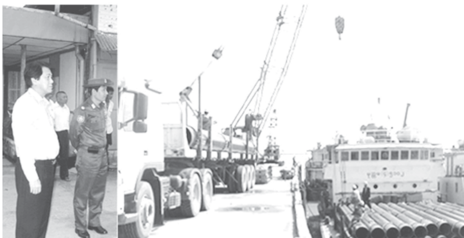
Deputy Minister Brig-Gen Than Htay inspects loading of PE coated gas pipes onto Z-craft.—ENERGY
