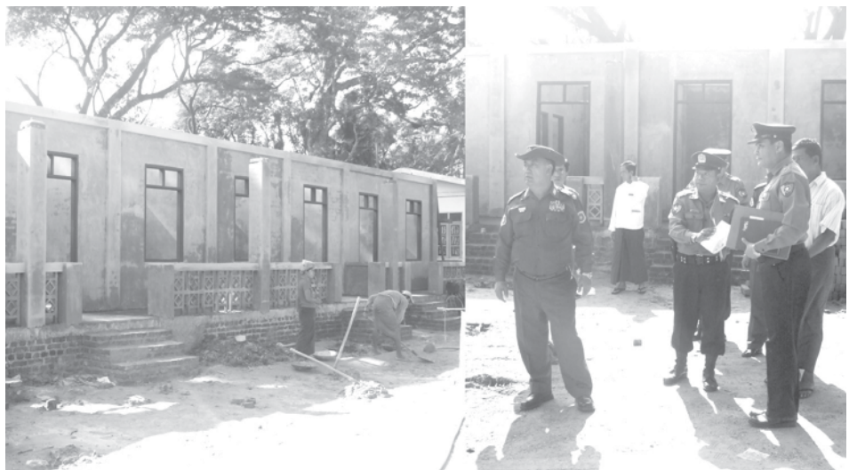
Minister Maj-Gen Maung Oo inspects construction of staff quarter in compound of police force in Nay Pyi Taw Tatkon Township.—MNA
