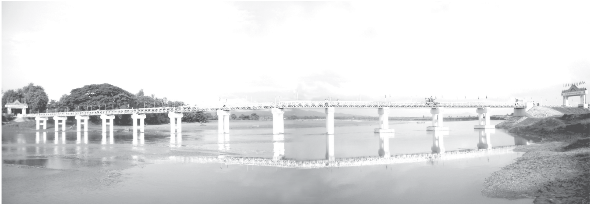
Photo shows newly-inaugurated Mindon creek bridge (Yenantha). CONSTRUCTION
