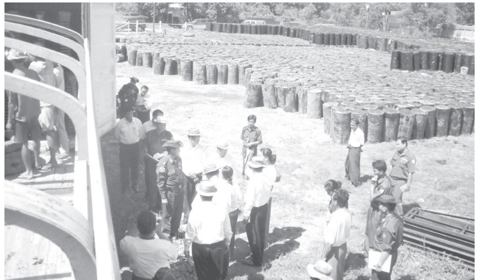
Minister Maj-Gen Khin Maung Myint inspects tar at storage and distribution department (Pynmabin) of Public Works.—MNA
