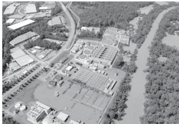
Floodwaters engulf parts of the RM Clayton Sewage Treatment Plant in Atlanta, Georgia, in this aerial view taken on 23 Sept, 2009.—XINHUA
