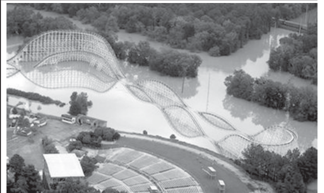
A roller coaster at Six Flags of Georgia Amusement Park is flooded on 24 Sept, 2009 in Austell, Ga. Several days of heavy rain has flooded parts of the Atlanta area.
