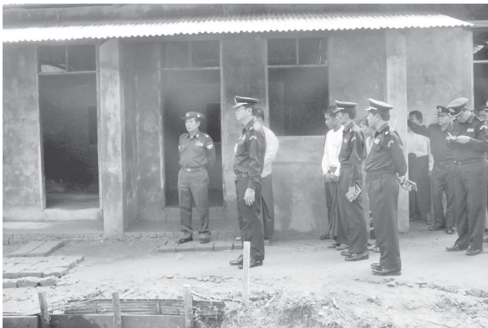
Minister Maj-Gen Maung Maung Swe inspects construction of fire station and staff quarter in North Okkalapa Township.—FSD
