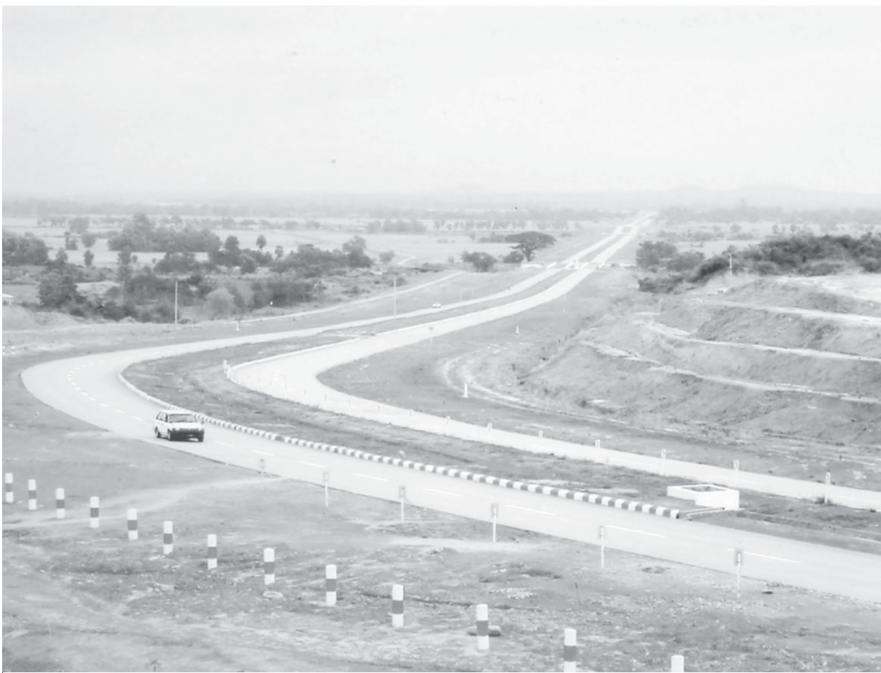
Nay Pyi Taw-Yangon road section of Yangon-Mandalay Expressway.
