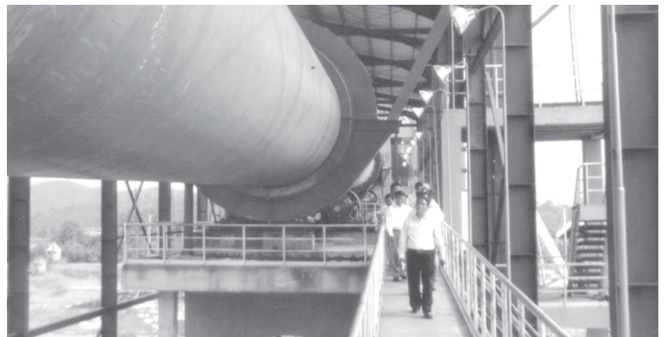
Minister for Industry-1 U Aung Thaug inspects 500-ton Nay Pyi Taw cement plant project (Taungphila).—INDUSTRY-1
