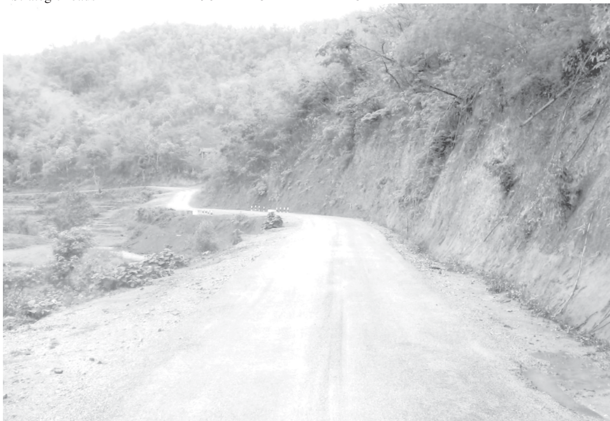
Photo shows Takaw-Mongping-Kengtung motorway in border region.
