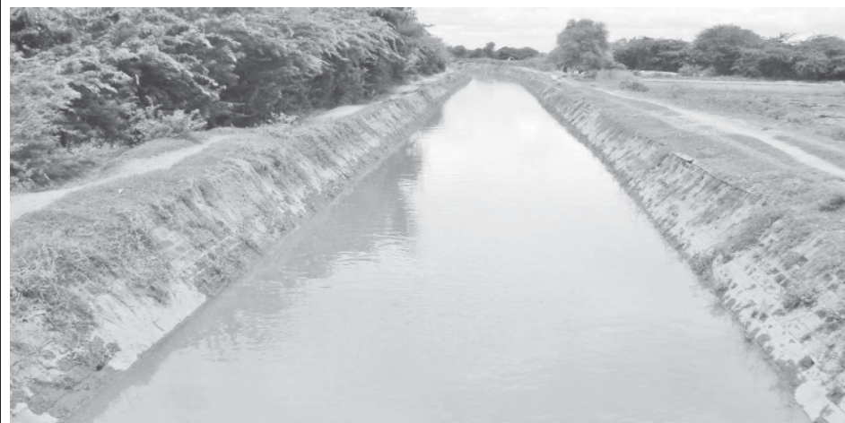
Paddy fields are irrigated through tributary canals of Thaphanseik Dam.
