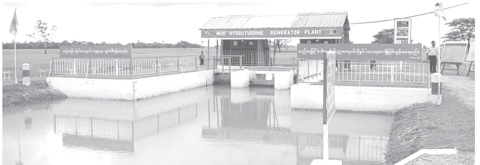
Photo shows Mini Hydro-turbine Generator Plant at Bogyigon Village in Thayawady Township.—MNA
