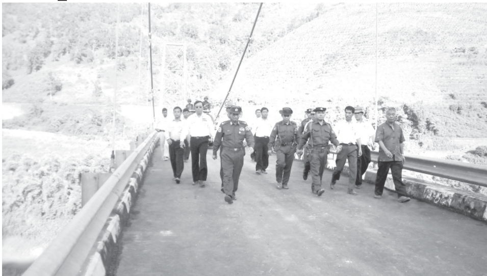
Minister Maj-Gen Khin Maung Myint viewing maintenance of Thanlwin Suspension Bridge (Tarpa).—CONSTRUCTION
