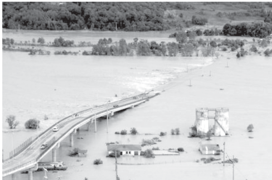
A bridge is partially submerged in flood in Istanbul, Turkey, on 8 Sept, 2009. Flash floods triggered by torrential rains killed seven people in north-western Turkey on Tuesday and three others were still missing.—XINHUA
