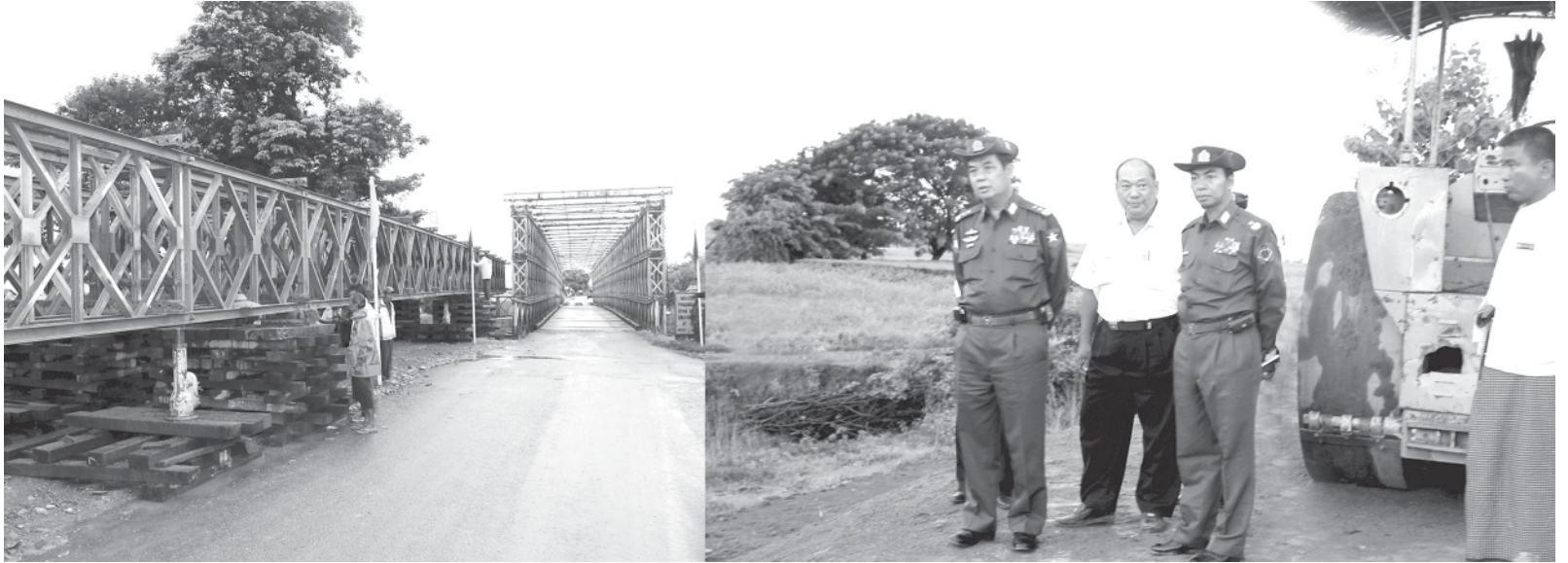
Lt-Gen Tha Aye of the Ministry of Defence inspects the construction project of Phaungku Bridge in Kale Township.
