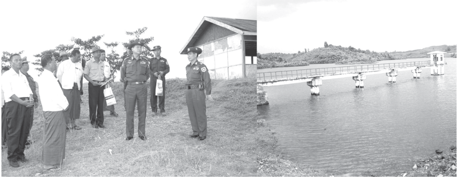
Lt-Gen Ko Ko of Ministry of Defence inspects supplying water from Hinywat dam in An.—MNA
