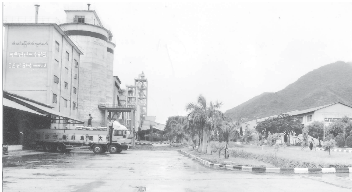
The compound of Cement Plant (Kyaukse).
