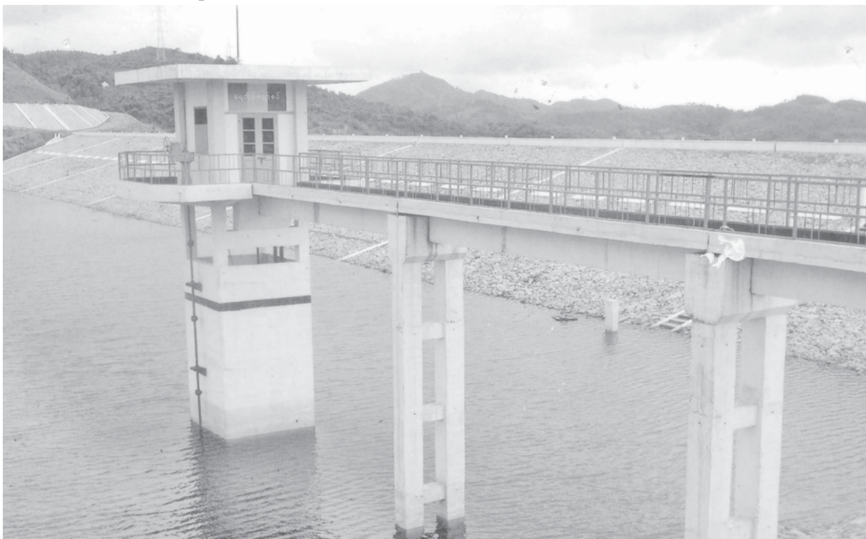
Control Tower of Sitha Dam.
