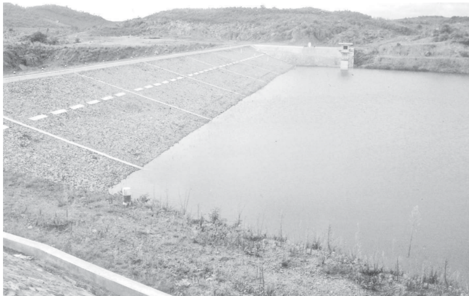
Water flowing into Sitha Supporting Dam.
