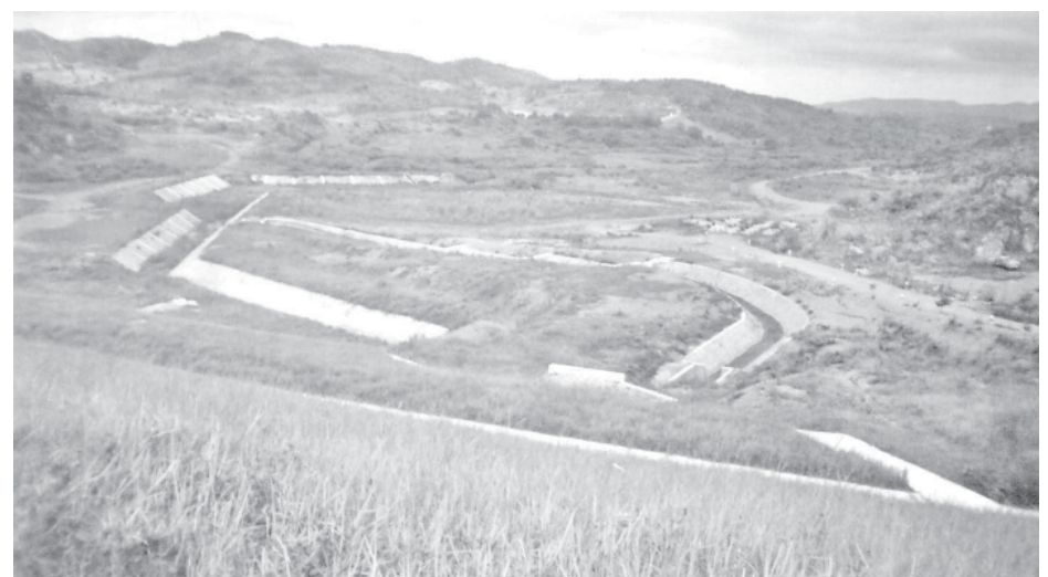
Sitha Supporting Dam providing water through concrete canals and pipelines.
