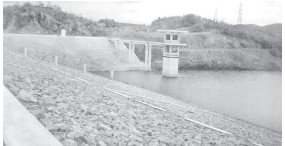
Sitha Dam alongside its control tower in PyinOoLwin Township, PyinOoLwin District.
