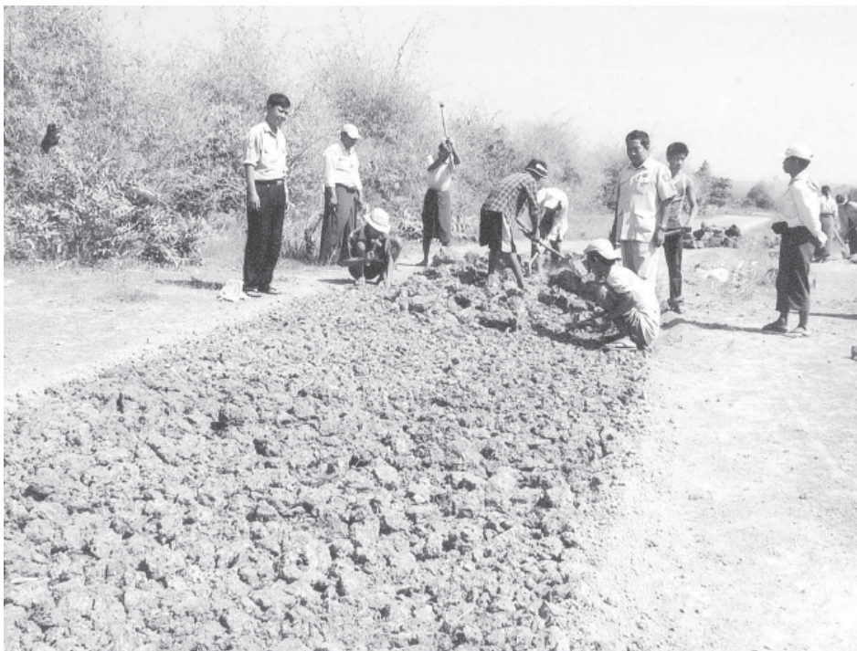
Building of Bago-Taungthusu village rural laterite road in progress.
