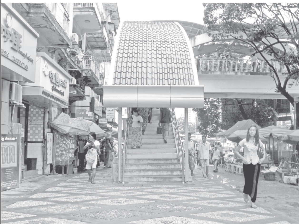
Tawwin Overpass seen on Sule Pagoda Road in Kyauktada Township.
