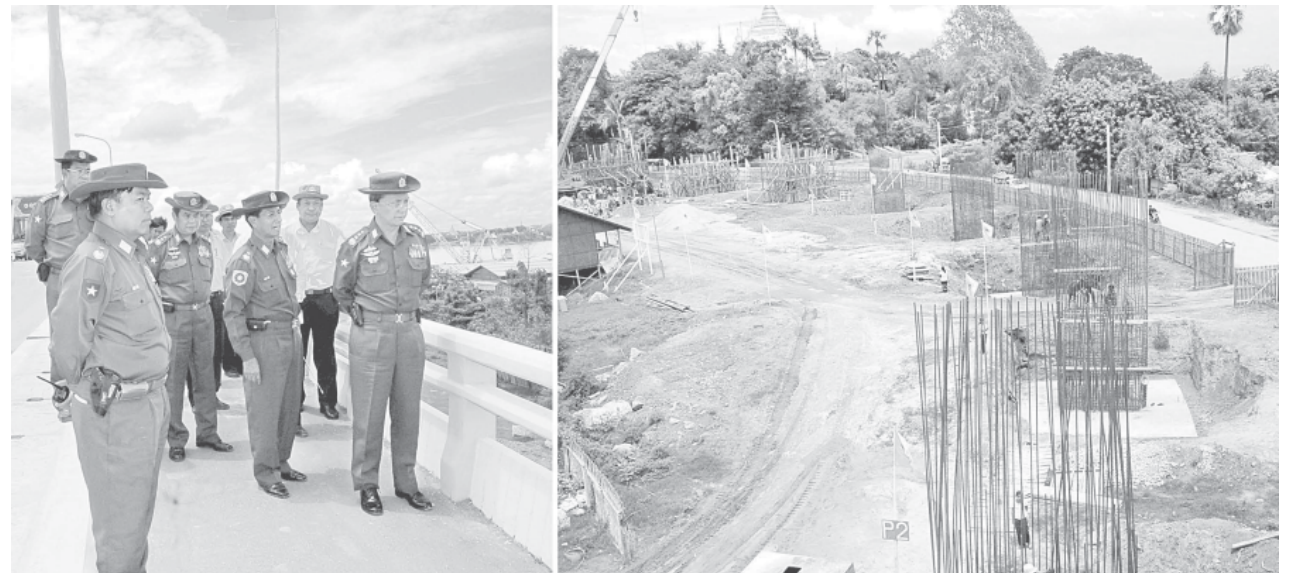
Prime Minister General Thein Sein inspects extended approach bridge of Ayeyawady Bridge (Yatanarpon) on Mandalay bank.—MNA
