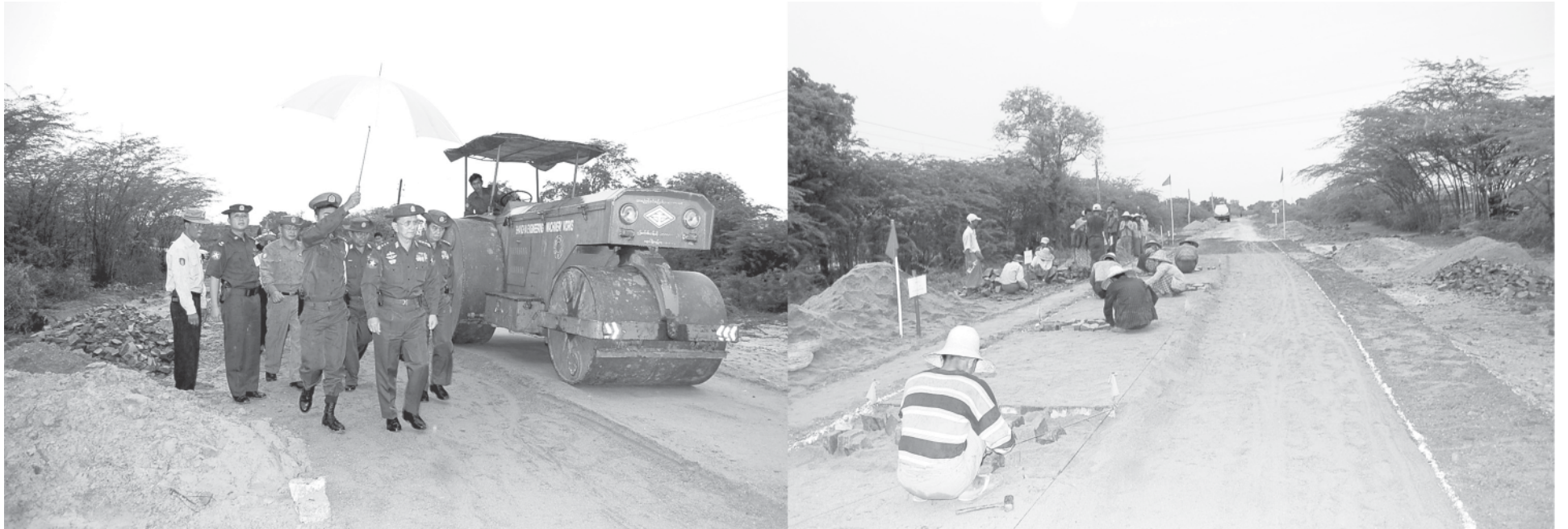
Prime Minister General Thein Sein inspecting construction of Thazi-Nyaungyan gravel road.—MNA
