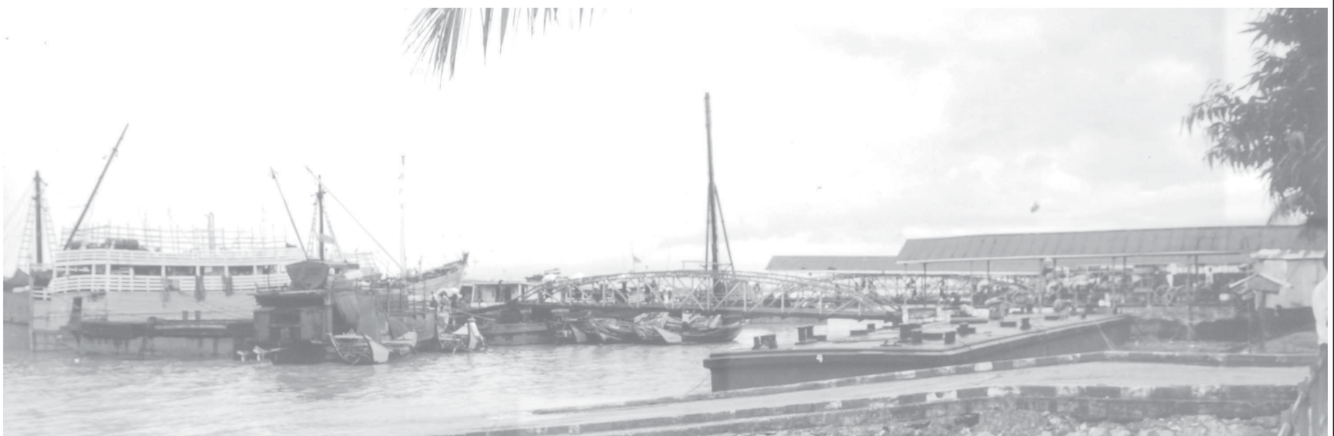
Wardan Pontoon Jetty No. 3 and Ro-Ro Ferry Jetty of Yangon Port.
