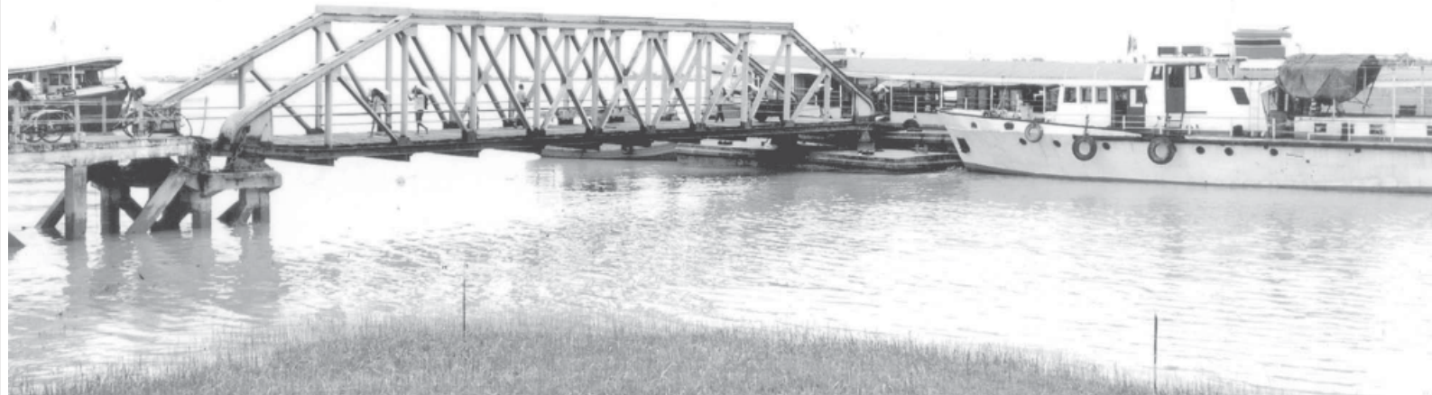
Cargo vessel from Bogale seen at Botahtaung Pontoon Jetty No. 5 of Yangon Port .
