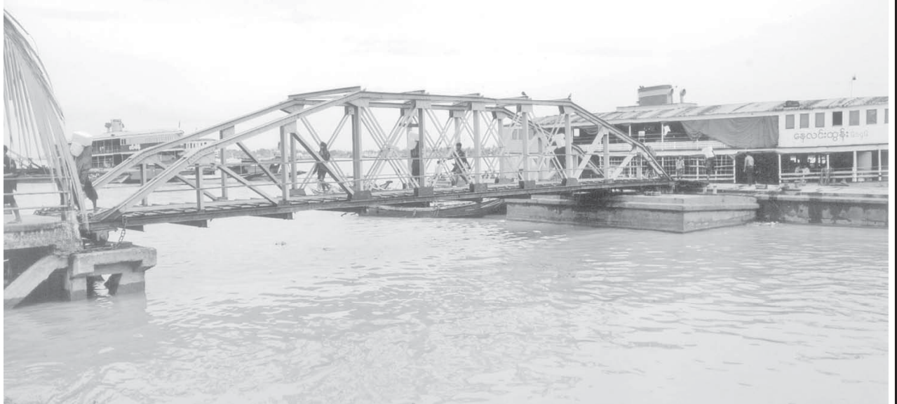
A ferry named Nay Lin Tun docking at Sinh-oh-dan Pontoon Jetty-1.
