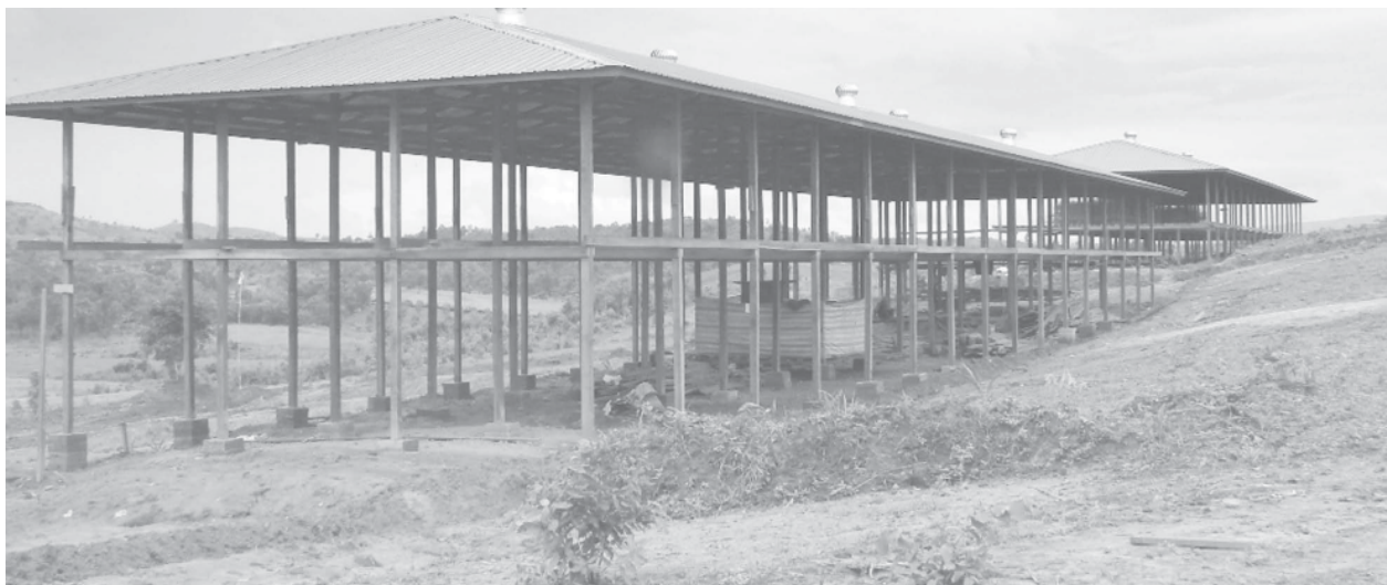
Construction of a chicken farm in Livestock Breeding Zone in progress.
