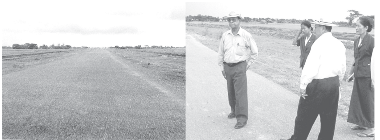
Deputy Minister U Tint Swe inspects approach road of Dagon Bridge.—CONSTRUCTION
