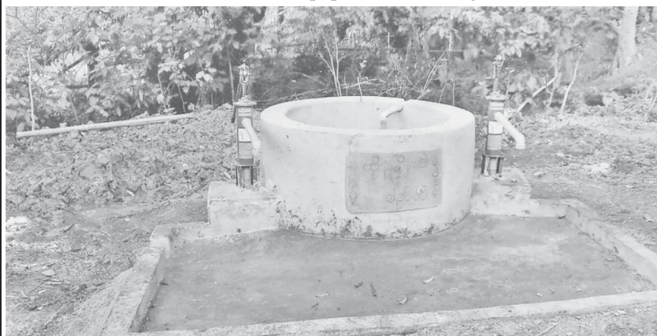
A manual pump in Kant-bein Village, Paunglin Village-tract.
