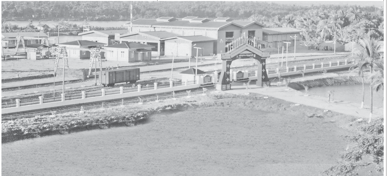
Mawlamyine Railway Station and Mottama Sleeper Factory.
