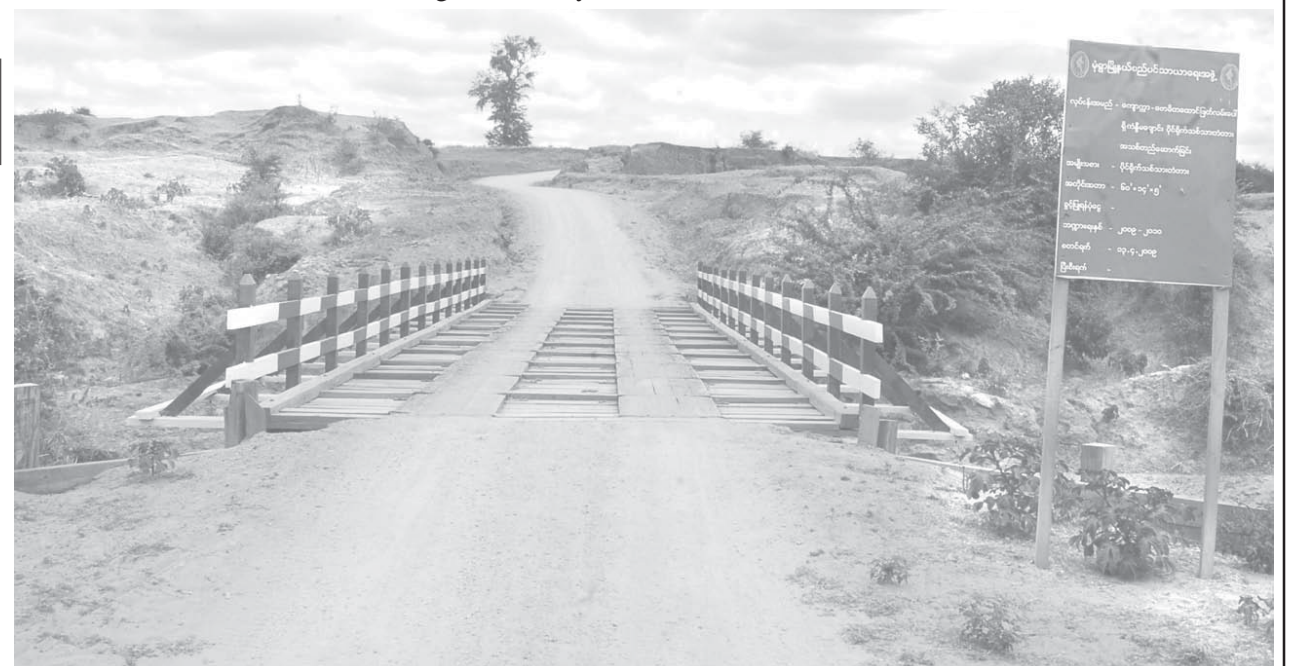
Kandima Creek bridge on Kyaukka-Bodhi Tahtaung shortcut.
