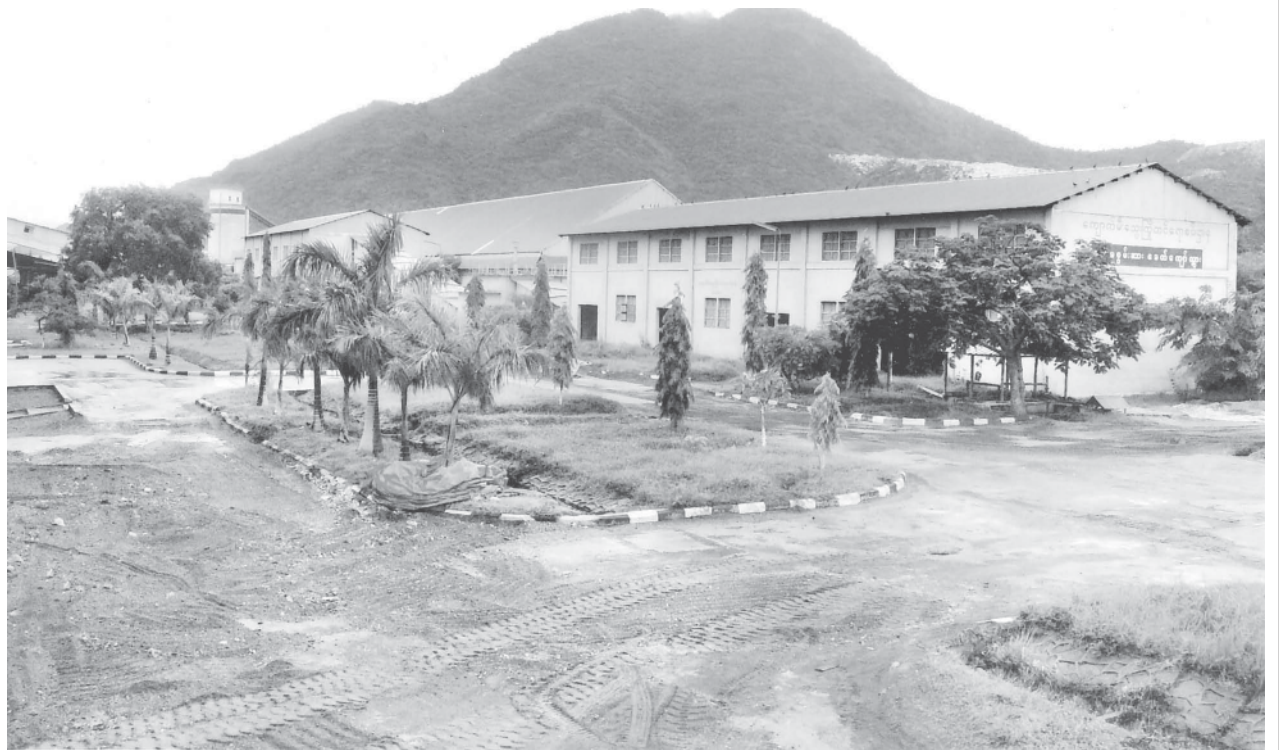
Cement Factory (Kyaukse) in Kyaukse Township seen with Mt. Thantawmyat in the background.
