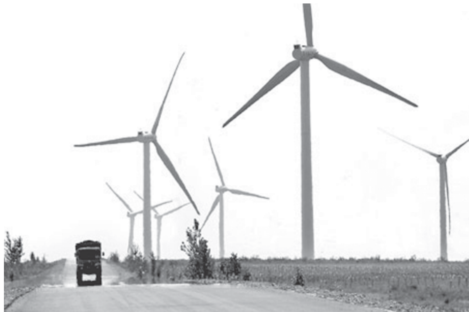
Huge turbines of wind power plants are pictured in Hinggan League (or prefecture) of north China's Inner Mongolia Autonomous Region on 7 Aug, 2009. Inner Mongolia, covering 1.18 million square kilometers of land, has boasted more than 3 million kilowatts of wind power, the largest of its kind in China. —XINHUA
