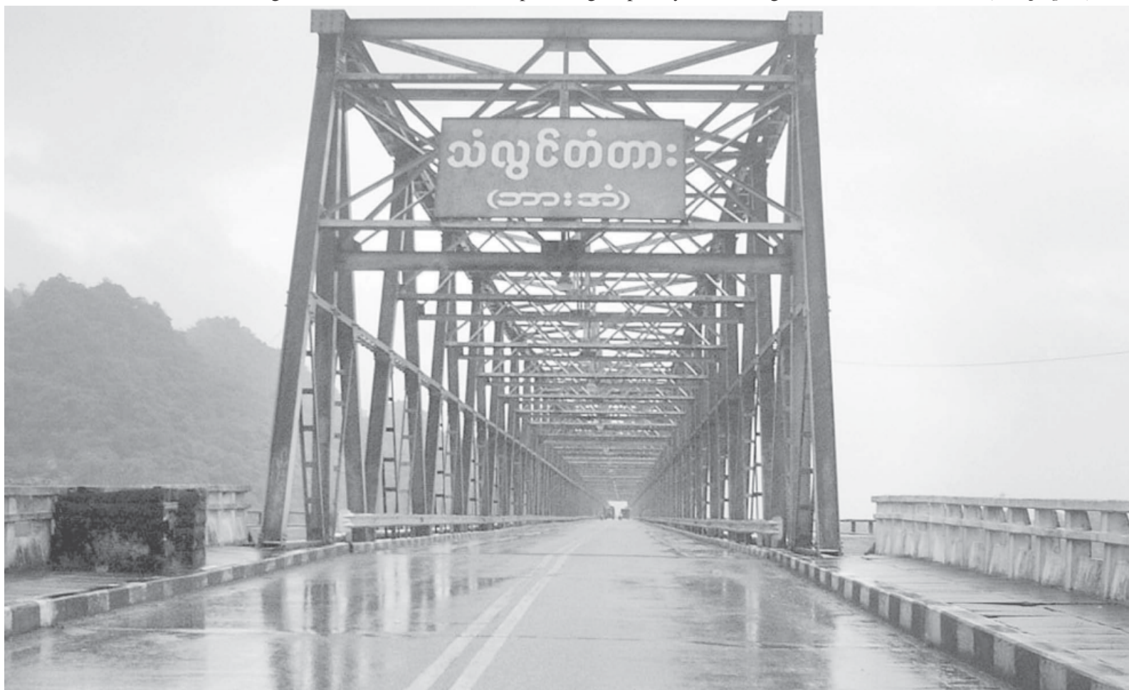
Thanlwin Bridge (Hpa-an) spanning the Thanlwin River.
