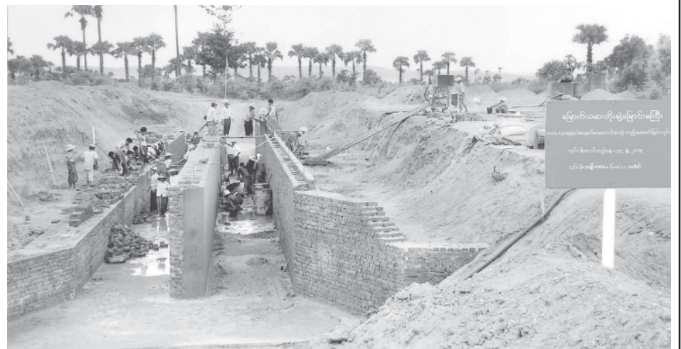
The drainage structure of the main canal is under construction.
