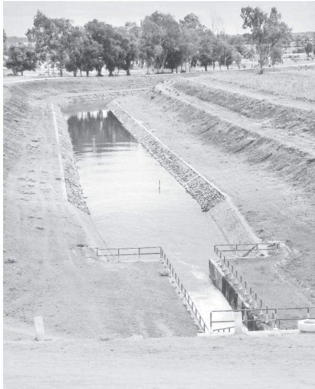
The intake structure of Myaukyama Irrigation System designed to irrigate 7500 acres of farmlands.
