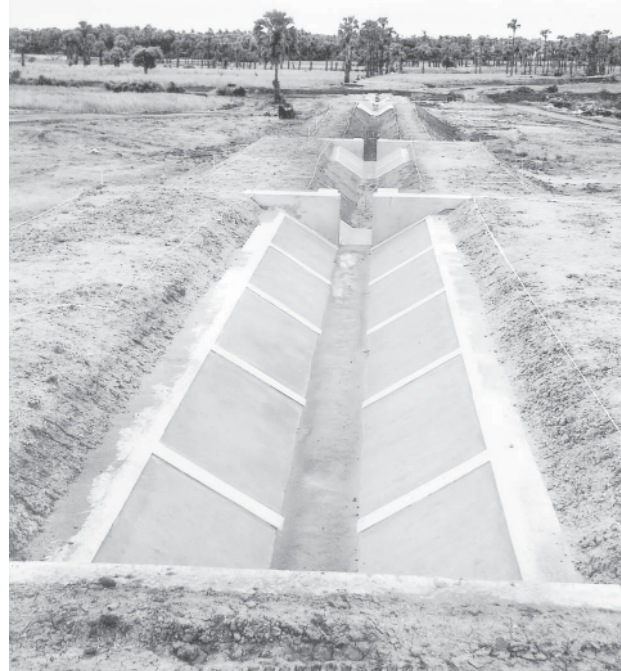
The intake structure of distributary (2) under construction.
