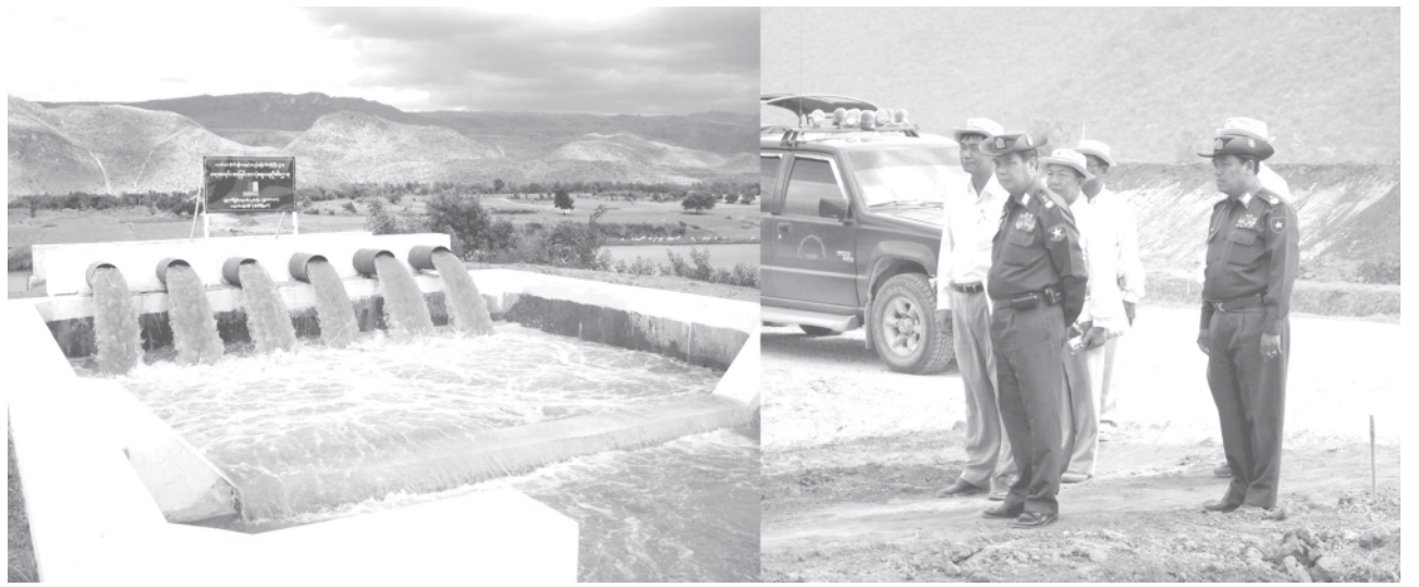
Lt-Gen Tha Aye of the Ministry of Defence looks into the progress of water pumping and water tank in Duhtawadi Water Pumping Station.—MNA
