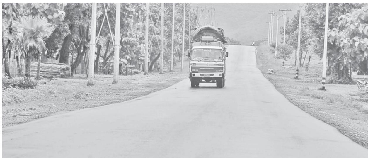
The already upgraded Bilin-Kyaikhto road section.
