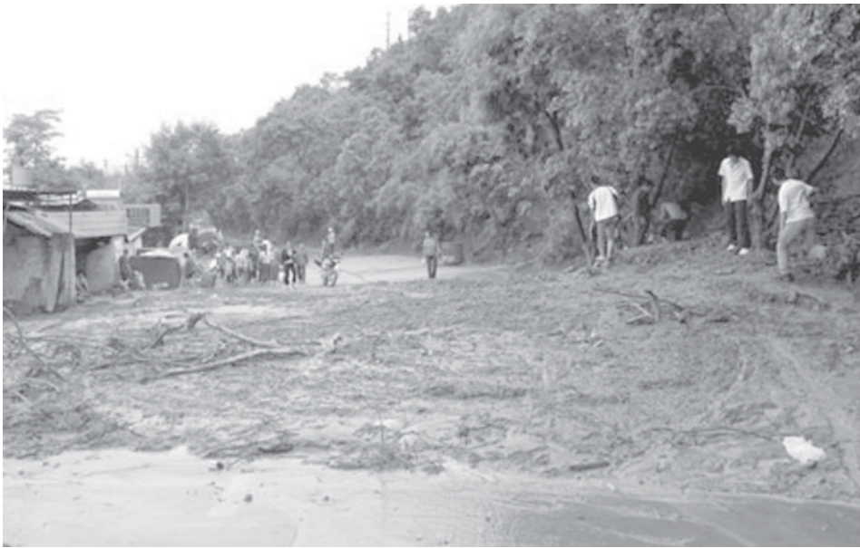
Photo taken on 27 July, 2009 shows the provincial road 214 damaged by the mudslide at Miyi County, Panzhihua City, southwest China's Sichuan Province. Twenty-two people are dead and seven missing after torrential rains triggered floods in Miyi County, local authorities said Monday.—INTERNET
