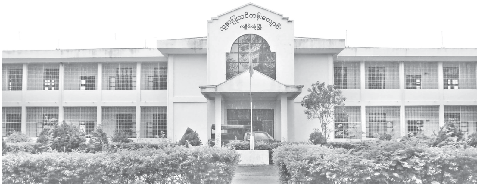
Photo shows two-storey RC building of Kengtung Nurses Training School.
